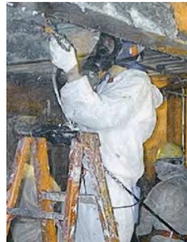
Removing asbestos fireproofing is tedious and requires significant manpower. Above certified asbestos abatement workers remove fireproofing from inside a negative pressure containment.
