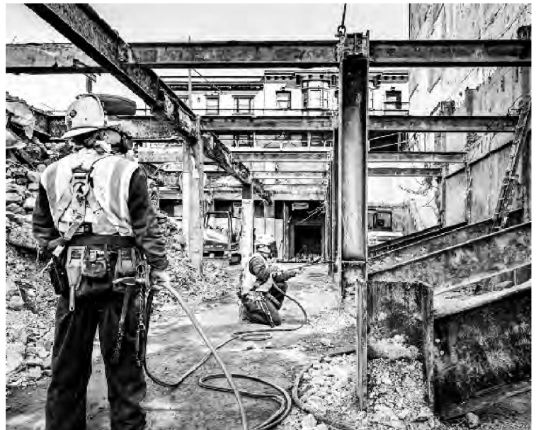
Above, Silverado manually isolates structures to protect buildings to remain. Similar efforts are required at the Harris and Enterprise Buildings as these buildings are separated from Carousel Mall.
